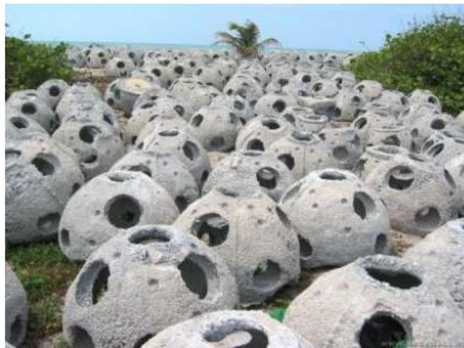
**Figure 4.17: Reef Balls before deployment (Source: Reef Ball Foundation, <http://www.reefball.org>)**
